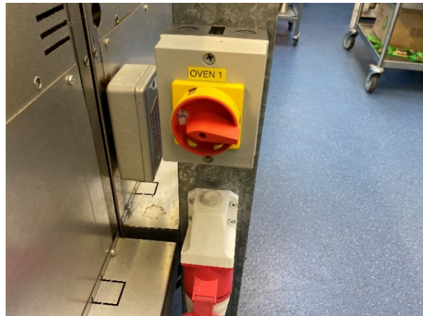
Electric ranges with isolation switch
