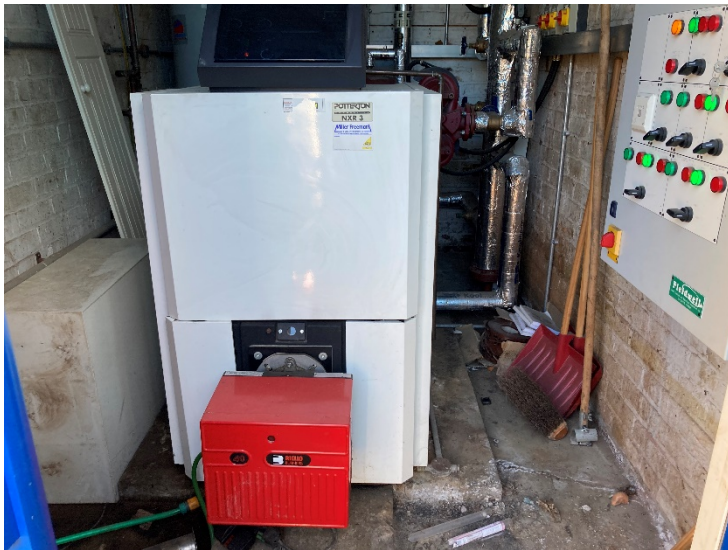
Single oil boiler
